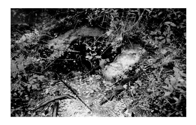
Figure 3. Photograph of the springhead, looking north (2000). The upper part of the concrete shaft surrounding the springhead has deteriorated on its south side.
